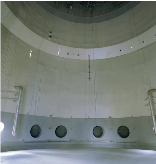
Absorber lined with COROFLAKE 24 and LINING 65 W
