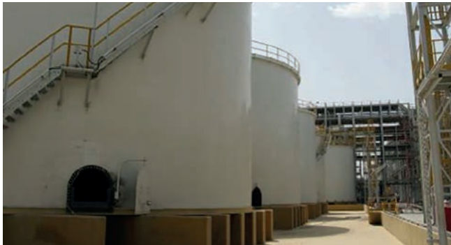
Coated secondary containment
