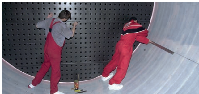
Lining of a filter tank
