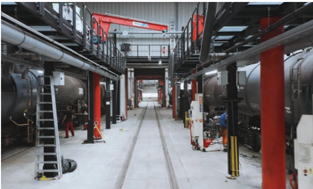
Kesselwagenhalle in Wittenberg
