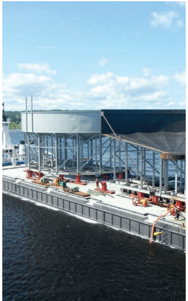
Delivery of rubber-lined thickener parts
