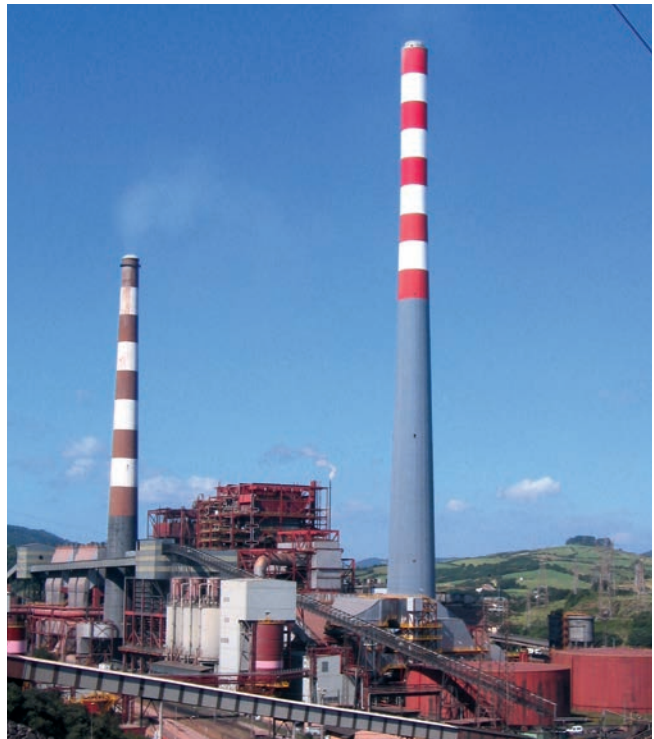
Coated power station chimney
