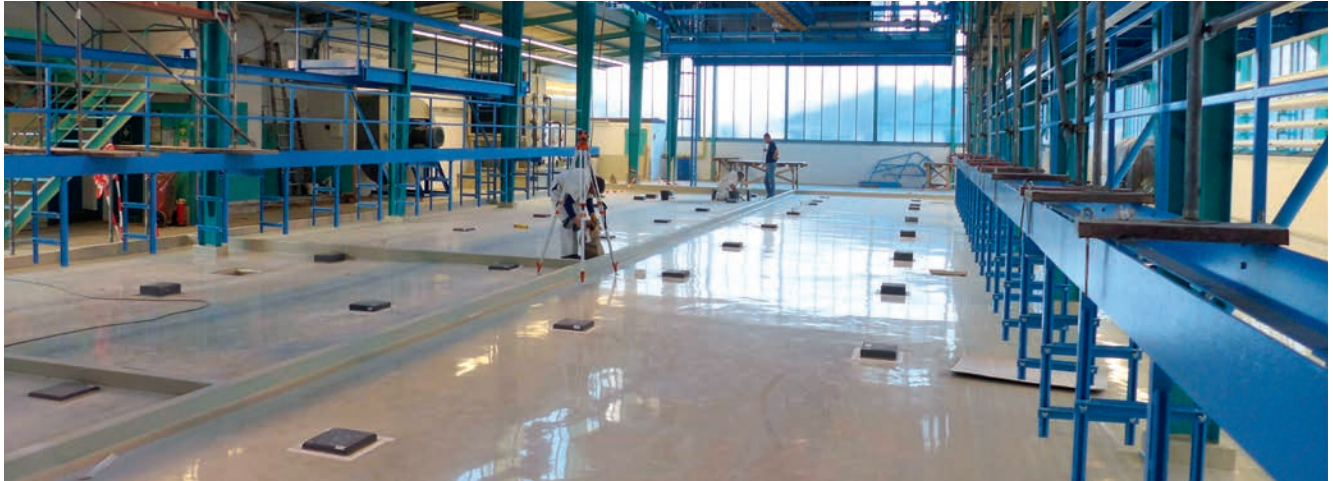
WHG coating of an impounding basin in a galvanizing facility
