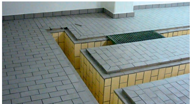
Combined covering implemented with gutters
