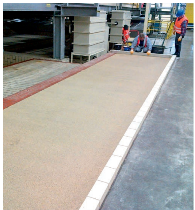
Installing a screed coating
