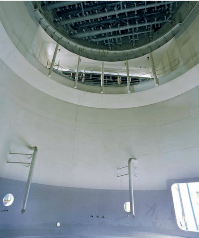
COROFLAKE coating in an absorber
