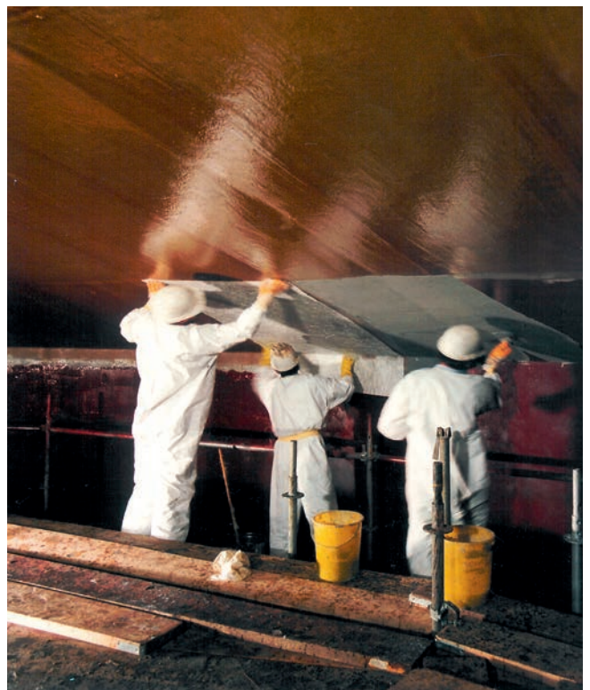
Installing a laminate coating
