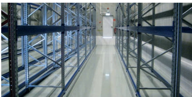
WHG coating in a shelf storage warehouse
