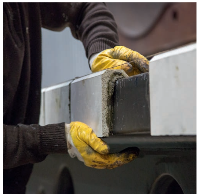
Working with synthetic resin mortar
